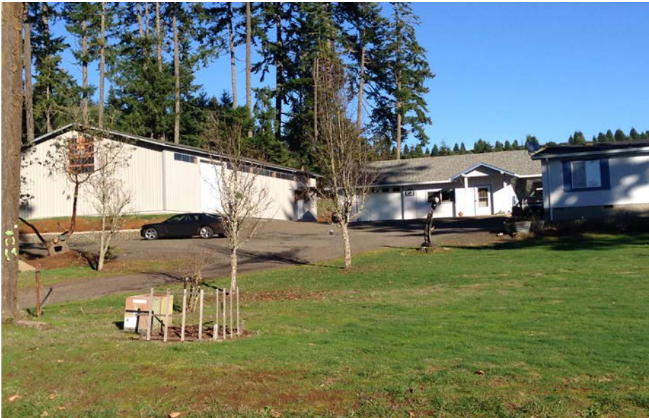
Photo 3: Heppel, C. (Photographer). (2014). Building compression . [Photograph].
