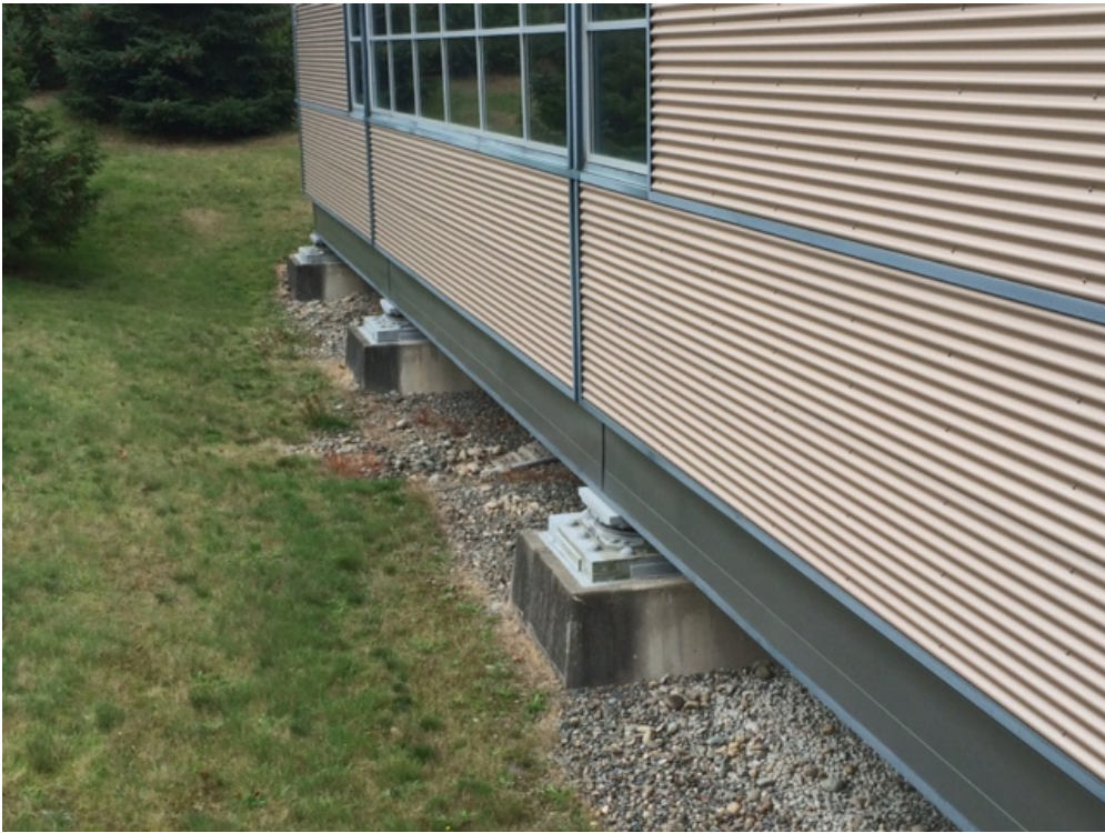
Exterior photo showing building foundation built for stability during an earthquake
