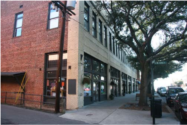
Lafayette Place, 200 South Lafayette Street
