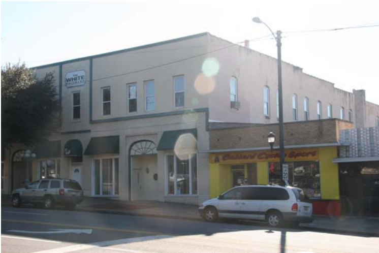
The White Building, 119 East Marion Street
