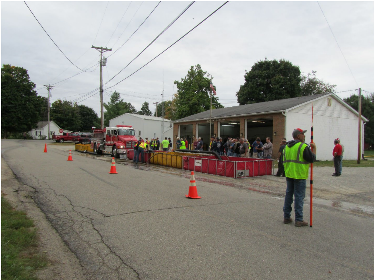
Figure 12. Traffic control at a dump site operation.
