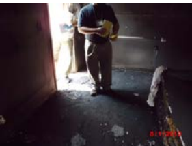
Lower southwest wall
