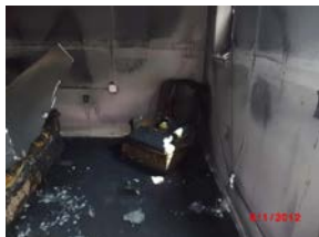
Lower southeast wall
