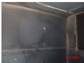
Upper northwest wall
