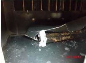
Lower northwest wall
