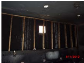
Upper north wall
