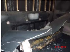
Lower northeast wall
