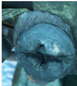
After fire exposure
