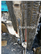
Post-fire photographs of non-fire-rated steel door and door frame.
