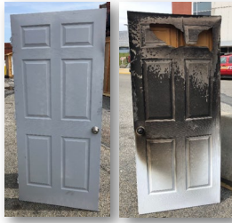
Post-fire photographs of hollow core door.
