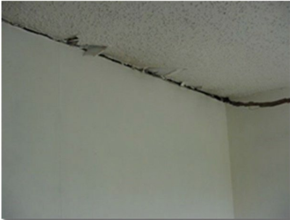
Image 2: pushing of ceiling/roof from fuel/air explosion.
