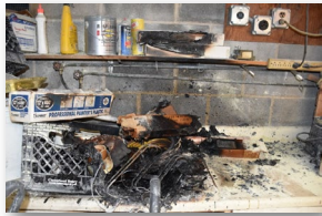
Small countertop fire
