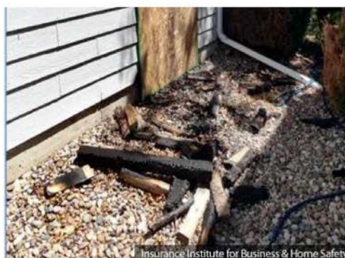
Figure 12: Embers ignited a firewood pile located next to the garage of this home. The direct flame contact exposure from the burning firewood ignited the composite wood (hardboard) siding product. Source: IBHS.
