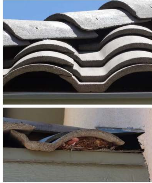
Figure D17: The ends of the barrel-tile roof covering on this home were not “bird-stopped.” Note the debris in the under-roof area at the end of the roof (lower photograph). Source: IBHS.
