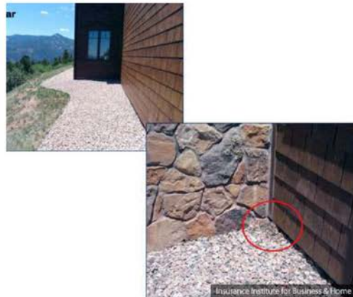
Figure D5: The upper left photograph depicts the vegetation management (defensible space) at the rear of the house. The lower right photograph shows an accumulation of dried vegetative debris in the corner, on top of the rock mulch. Source: IBHS.
