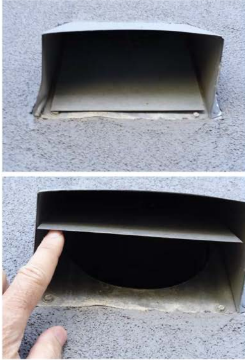
Figure D24: Dryer and other exhaust vents used vents coverings that were normally closed (upper left); when operating positive pressure in the duct would force open the closure flap to at the outlet. Source: IBHS.
