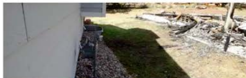
Figure 11: The distance between the destroyed home on the left and the damaged home on the right was approximately 16 feet. Source: IBHS.
