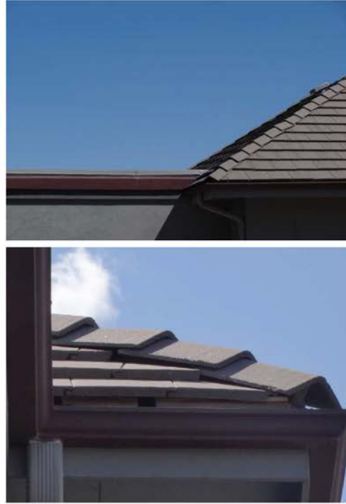
Figure D25: A flat concrete tile was used for the roof covering on this house. Note the openings at the hip and edge of the roof. Source: IBHS.
