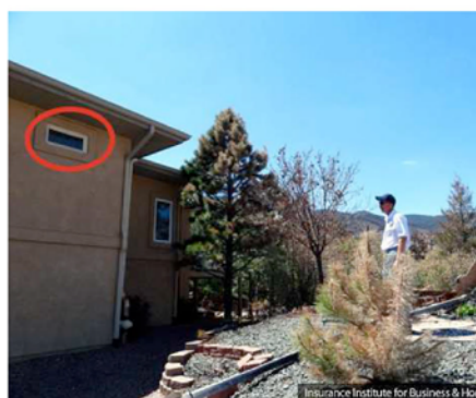
Figure 7: This damaged Talleson Court home was approximately 30 feet from a destroyed home. Two windows were damaged (one is circled in red; another window of the same size is located to the left of the one shown). The tall pine tree had lower branches removed and noncombustible gravel was used within approximately 10 feet from the house. Note the scorch on the destroyed home side of the pine tree and small tree in the foreground. Source: IBHS.
