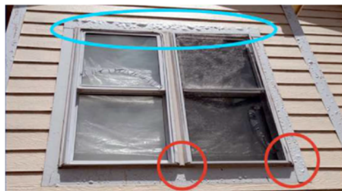
Figure 13: Radiant heat from the burning home, which was destroyed and was located 20 feet from this damaged home, was sufficient to cause paint on the wood trim to bubble (circled blue) and thinner components on the vinyl window frame to deform (circled red). Source: IBHS.
