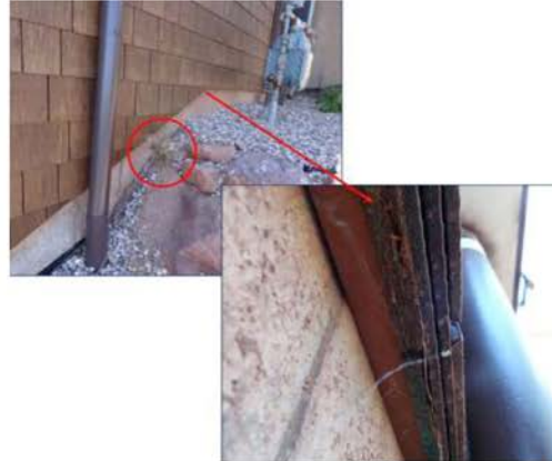
Figure D4: The upper left photograph depicts the vegetation management (defensible space) in the 0-to-5 foot zone on the left side of the house. The lower right photograph is a bottom-view of the wall construction consisting of oriented strand board sheathing under the fiber cement shingle siding product. Source: IBHS.
