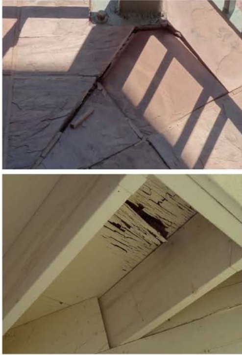
Figure D19: The flagstone covering on this solid surface (noncombustible) deck had failed (upper) allowing water to get below the covering, eventually resulting in fungal decay in the horizontal wood-based sheathing (lower). Source: IBHS.
