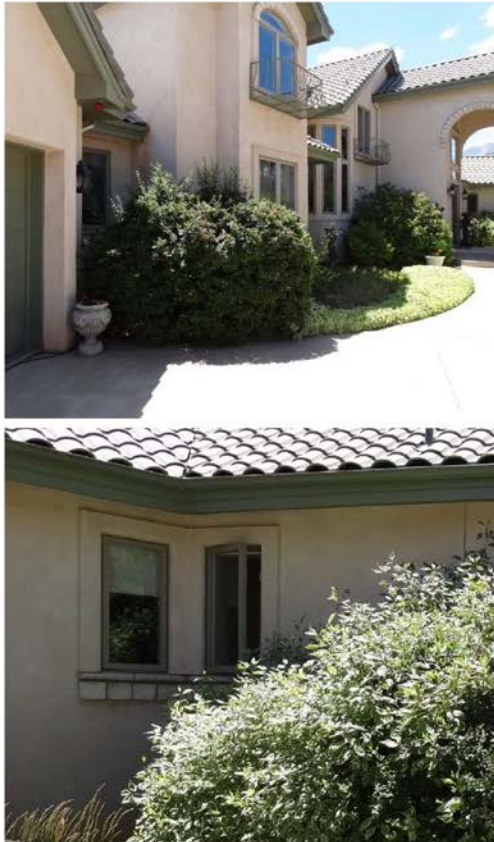
Figure D10: Near-home vegetation was prevalent at the front of this home. Note the open window in the lower photograph. Source: IBHS.
