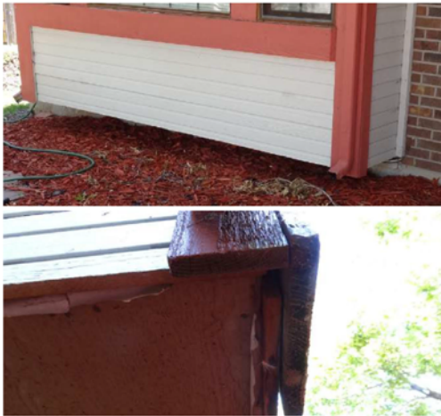
Figure 28: The "bump out" design feature at the front of the Rossmore Street home would be vulnerable, if the wood mulch had been ignited by the observed ember exposure. Given the low earth-to-wood clearance, flame spread to the bump out would have provided a flame contact exposure to the combustible underside feature. Source: IBHS.
