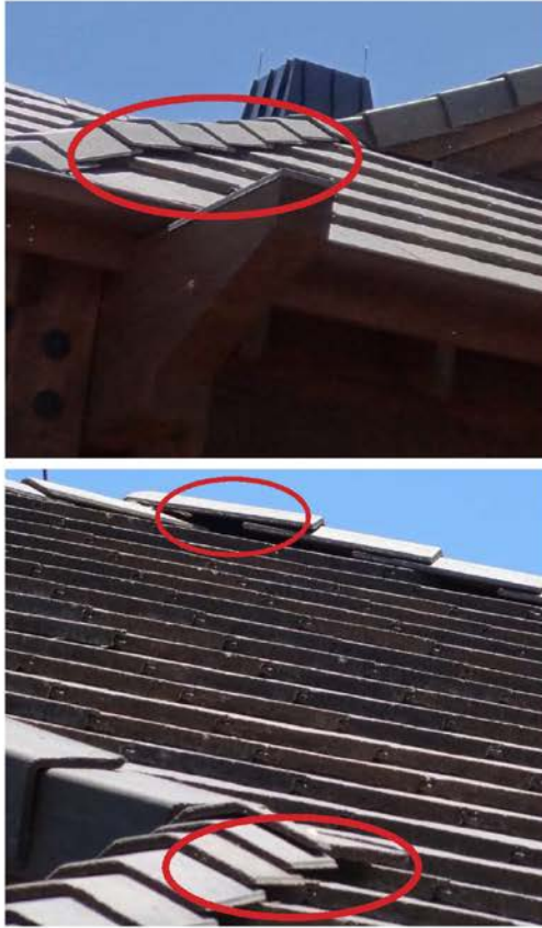
Figure D8: Un-stopped/unblocked openings at the hips of the flat-tile roof. Source: IBHS.
