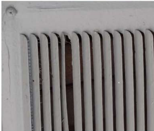
Figure D16: A soffited eave was used on this home. Some of the under-eave vents did not have mesh screening. Source: IBHS.
