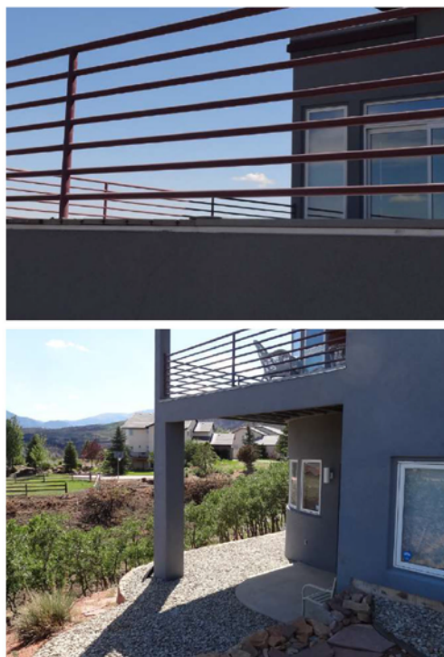
Figure D23: The decks at this home used wood for the structural support system and a combustible wood-plastic composite decking (walking surface) product. Source: IBHS.
