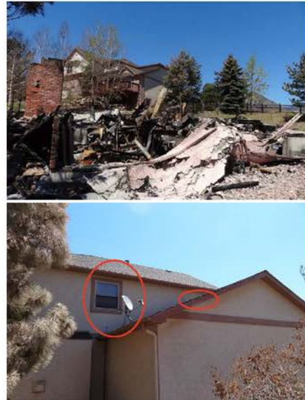
Figure 18: A composite figure of two damaged homes on the west side of Courtney Dr. The up-slope home is above and the down-slope home below. The charred combustible siding in the up-slope home is not visible in this figure. The damaged components in the down-slope home are circled. Source: IBHS.
