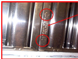
Directional arrows on filters
