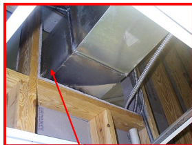
Improper clearance to the wood framing
